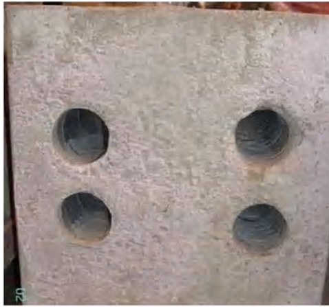
a ) Top column, showing corrugated sleeves to receive bottom column bars
