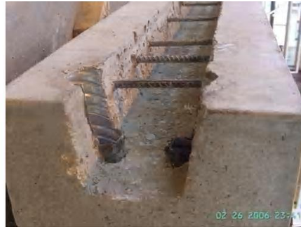
b ) Beam, showing the end at the connection side where sleeves are installed to bypass bottom column dowel bars
