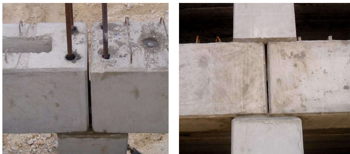
Figure 1.1 Discontinuous beam-column connection used in a braced frame car park project – Preconco Ltd., Barbados, 2010
