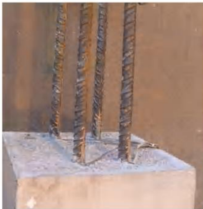
c ) Bottom column with 4H20 mm protruding bars
