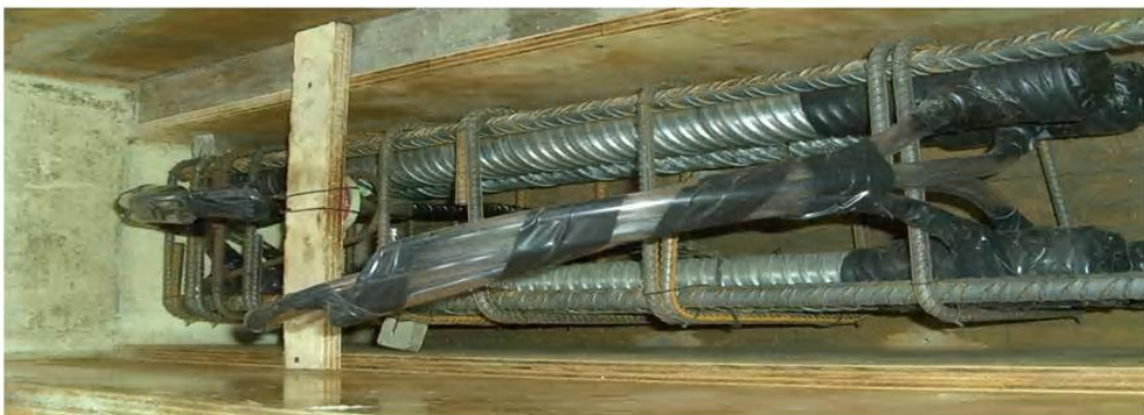
e ) Top column form work at the end that connected to the connection
